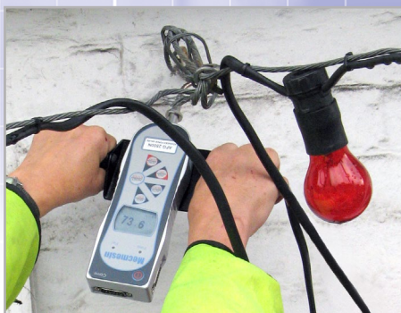
Pull test on anchorage points
