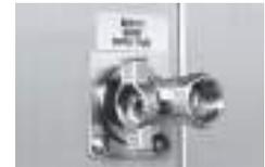
Pure water coupling (with pressure-reducing valve)
